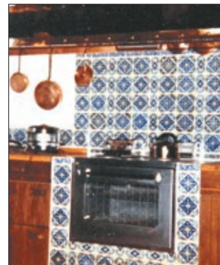
Monroe installed the yellow and blue tiles that frame the side of the kitchen stove.
